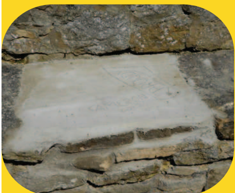
The seat after it had been repaired.
