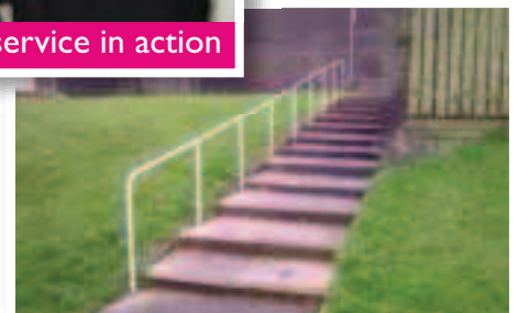
New handrail at Oakerside Drive
