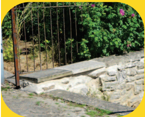
The wall after repairs.
