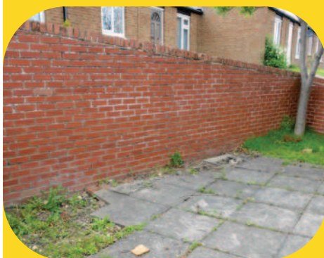
The bench has now been removed
